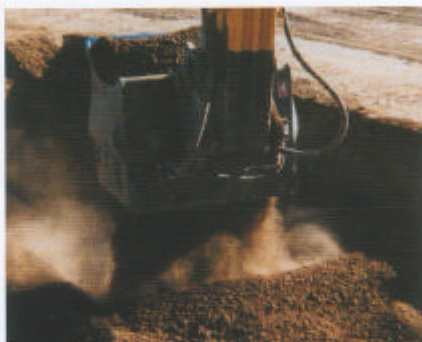
Screening rather than crushing protects against potential coating damage.
